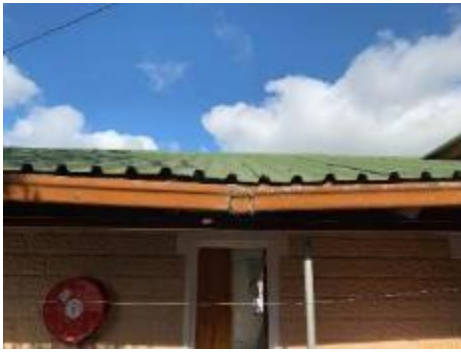
Broken gutters replaced with new aluminium gutters – thank you to Jon Lisher of AquaFlow.
