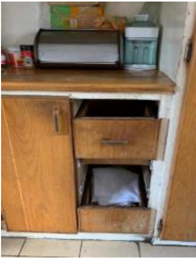
Kitchen cupboard doors repainted and repaired and new drawers installed.
